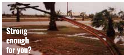
Figure 2: A Steel power pole bent by the wind strength of Tropical Cyclone Vance, 1999
